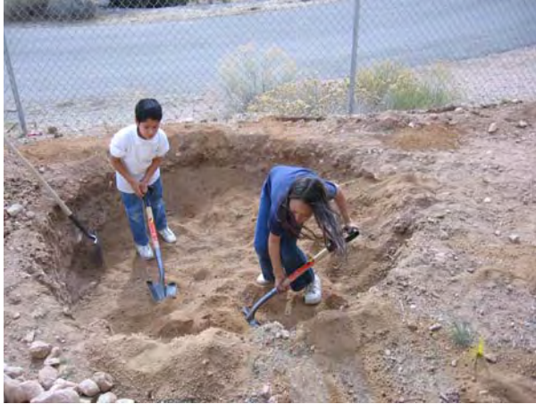
Students smoothing and leveling the base for the tank
